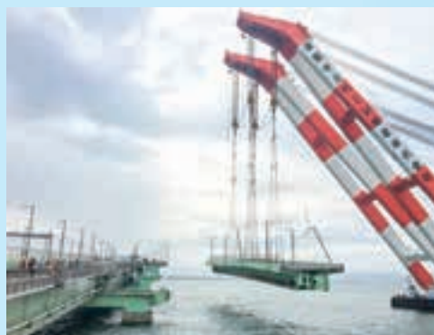
Removal status of damaged bridge girders
