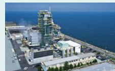
Biomass power generation plants
