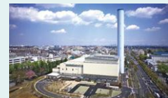
Waste-to-energy power generation plant
