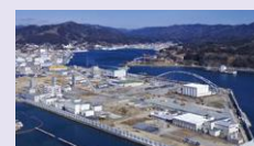
Hybrid tide embankments
