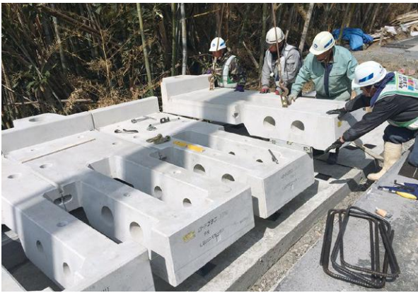
Precast concrete products for extending road width
