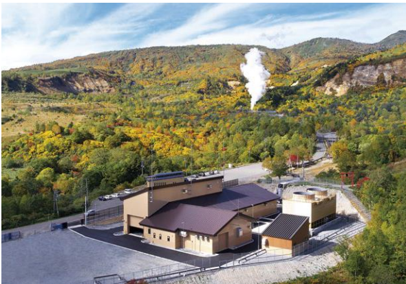
Matsuohachimantai Geothermal Power Plant operated by Iwate Geothermal Power Co., Ltd.
