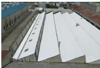
Roof with thermal barrier coating
