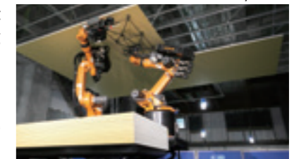
Robo-Buddy installing a ceiling
