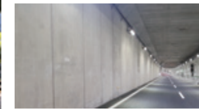
Labor/saving for construction of the "Large Section Box Culvert" by the "Hybrid Half Pre-casting Method": At the A-ramps for turn off of Keiyo Junction in Tokyo-Gaikan Expressway
