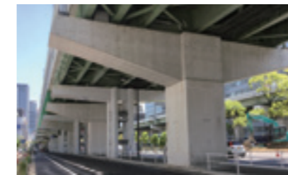
Widening method for urban expressway (Nishi-Semba Junction)
