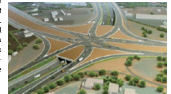
Tema IC Underpass construction to improve the intersection in Ghana (completed perspective)
