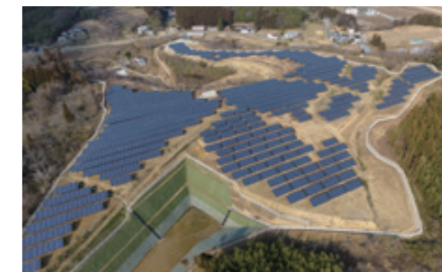
Solar power plant in Tome, Miyagi Prefecture
