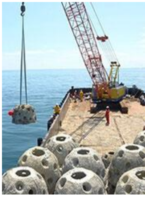
Installing artificial reef balls
