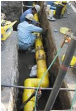
Replacing old pipes
