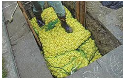
Gas pipeline installation work using Eco-balls
