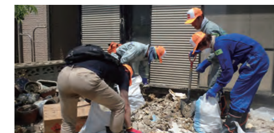
Rubble removal work
