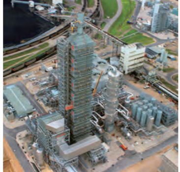
CO 2 recovery plant
