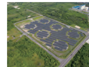
Kudamatsu Mega Solar Power Plant
