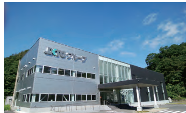
JXTG Group Safety Education Center
