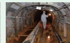
Gallery inspection at Hanawa Mine
