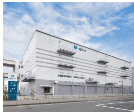
Logicross Yokohama Kohoku
