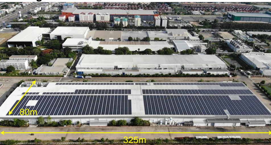
Bang Pa-in Plant
