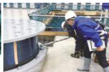
Confirming installation of a seismic base isolator
