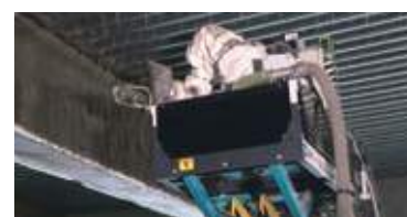
Construction using a fireproof coating spray robot
