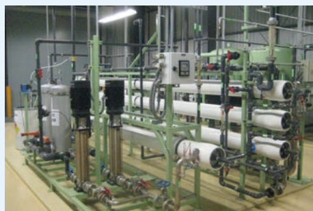
Filtration device using reverse osmosis membranes
