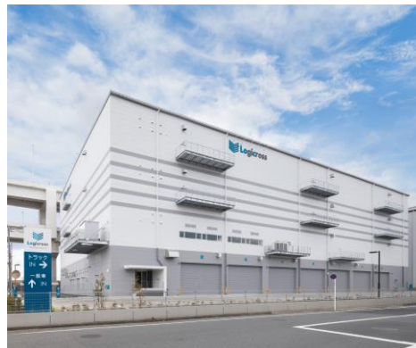
Logicross Yokohama Kohoku
